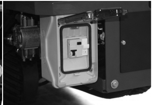
Fig. 143 Main supply switch
