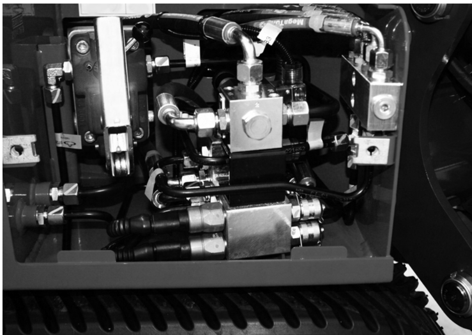
Fig. 165 Pressure check on the machine
